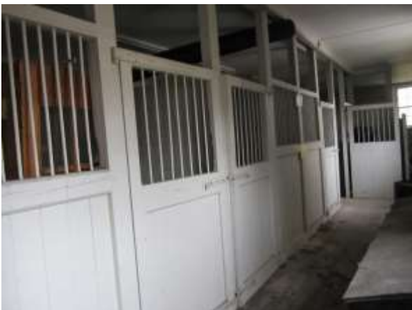
The stalls in the North block are in good condition
