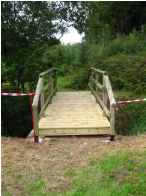
The new footbridge
