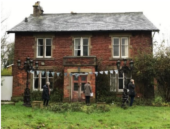
The farmhouse's Victorian Façade.
